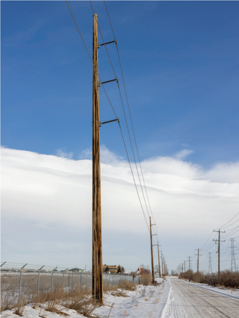
Example of Laminated Wood Pole
