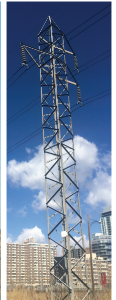
EXISTING LATTICE STRUCTURE
