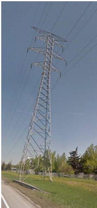
EXISTING TRANSMISSION STRUCTURE
