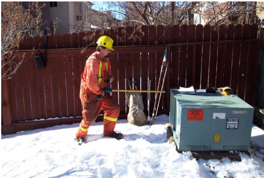
ENMAX program for testing transformers for PCB's
